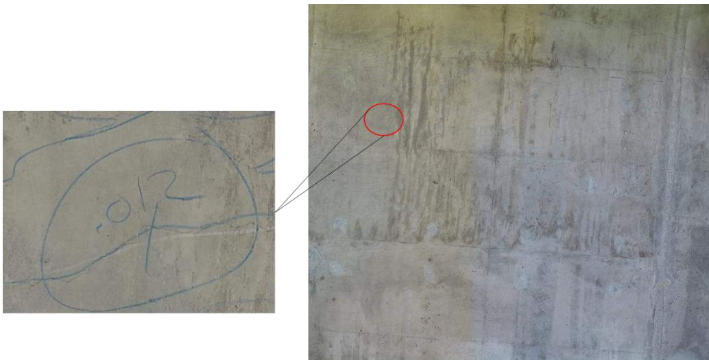
Figure 3.63: 2D Orthofacade of a Bridge Segment's Facade
