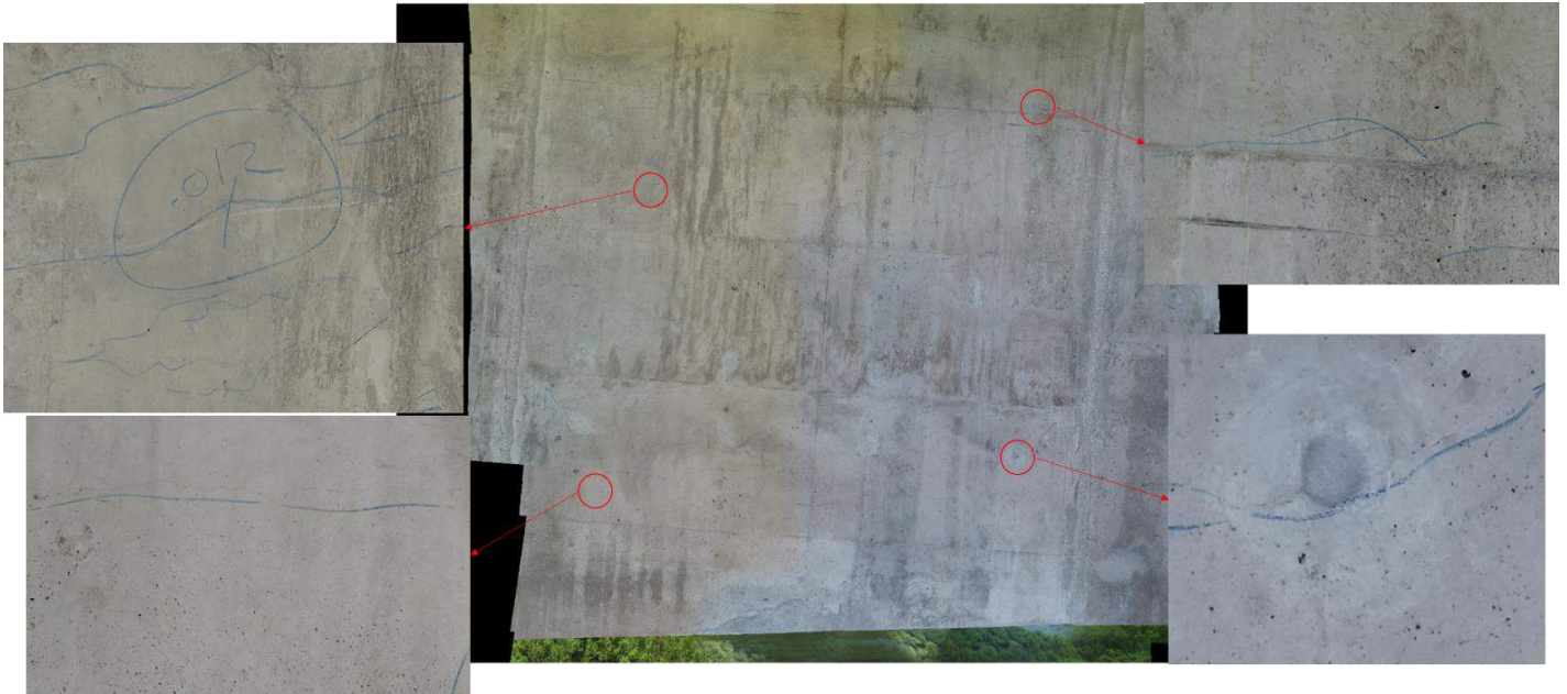
Figure 4.50: Pix4D Orthofacade of Segment P2-3D on the Southbound Bridge
