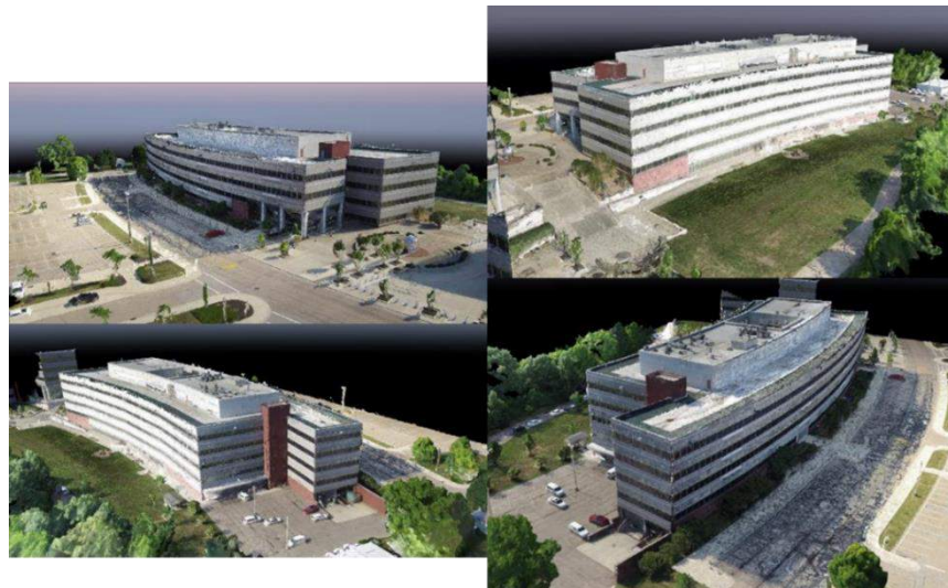
Figure 4.21: 3D Views of the 3D Point Cloud Generated Using the Visual Images of ODOT HQ
