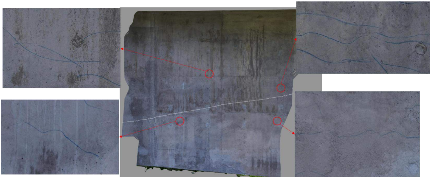
Figure 4.51: Context Capture Orthofacade of Segment P2-3D on the Southbound Bridge
